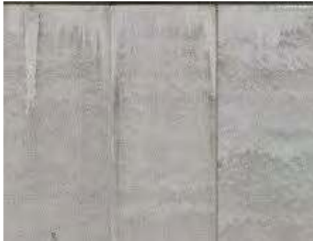
Off form Concrete
